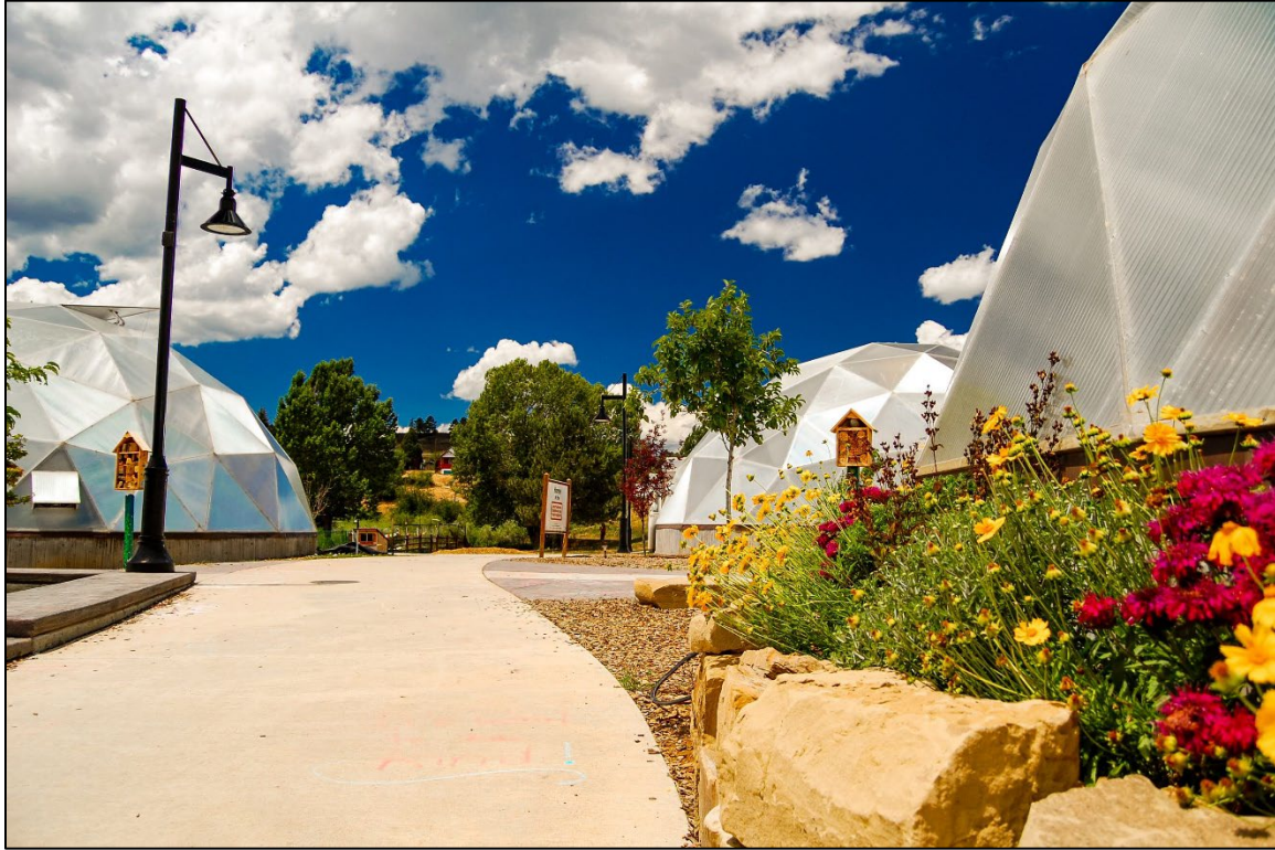
Geothermal Greenhouses in Centennial Park
