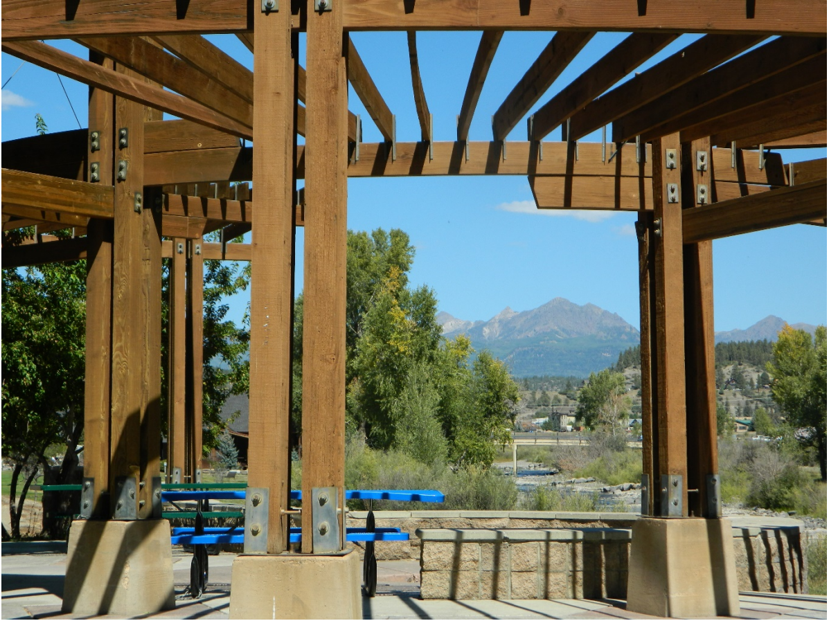
Terrazzo at Yamaguchi North Park
