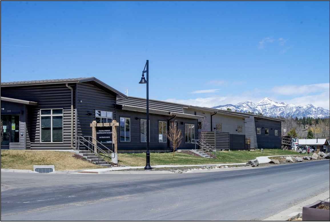
Town Maintenance Facility
