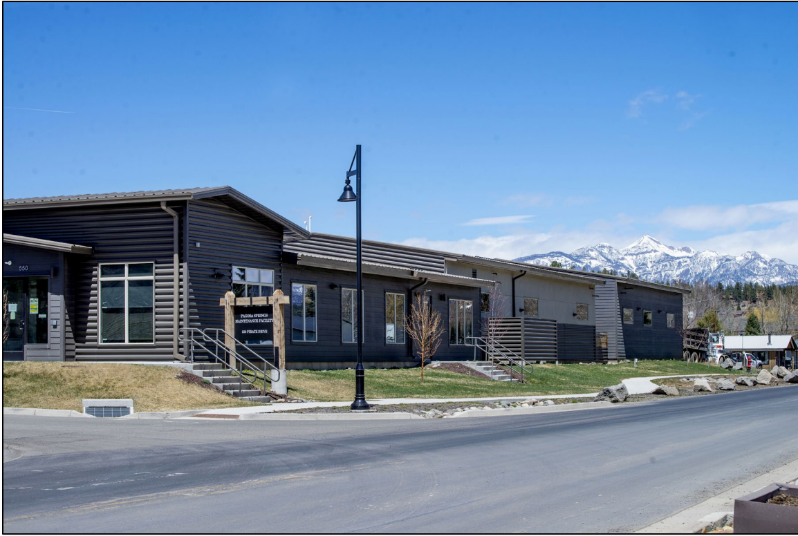
Town Maintenance Facility
